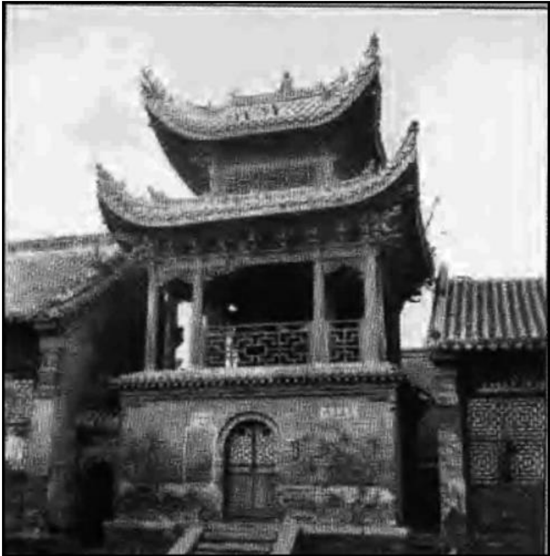
Figure 32 The stage of Shanshangan Hall in 1930.
