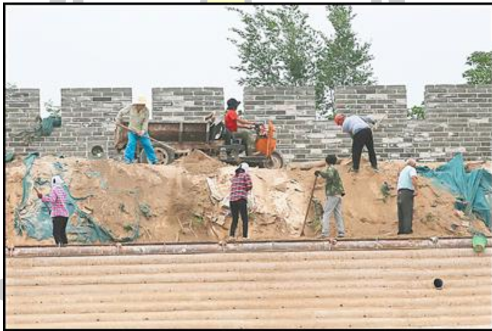
Figure 61 Restoration work of the ancient city wall
