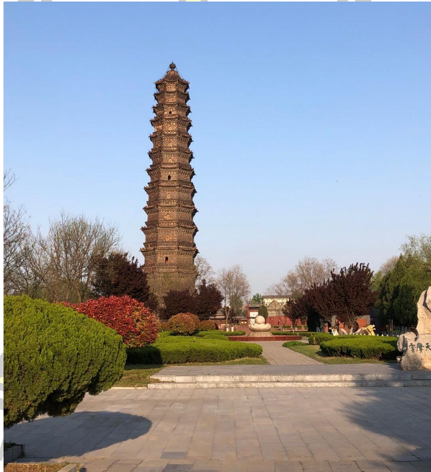
Figure 53 The iron tower park
