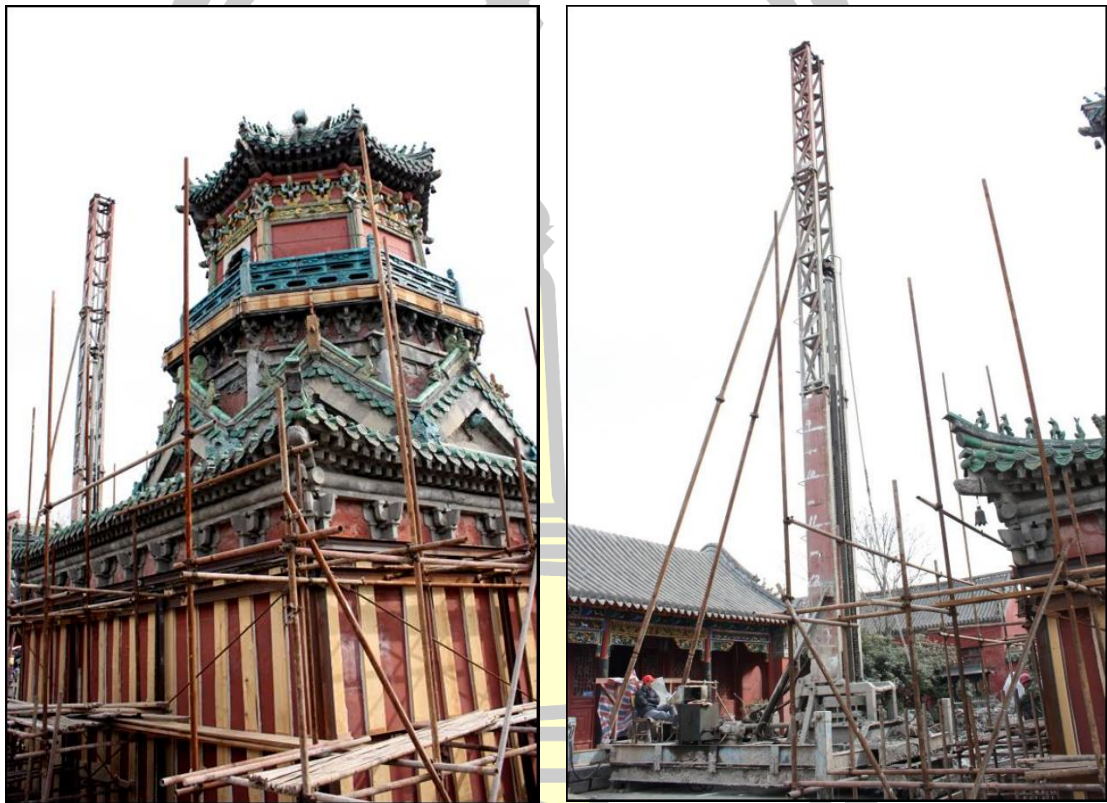
Figure 40 Construction process of the Yanqing Temple jacking project.
