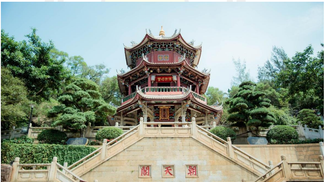
Figure 20 The Chaotian tower Source: Photographed by Ke Yihan, 2020
