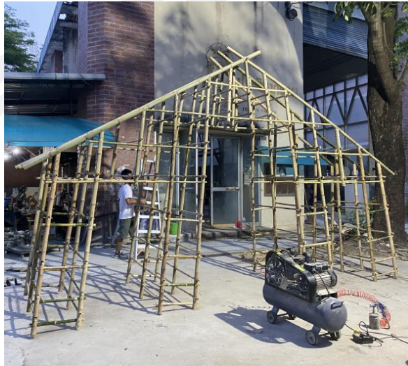
Figure 37 The frame is complete
