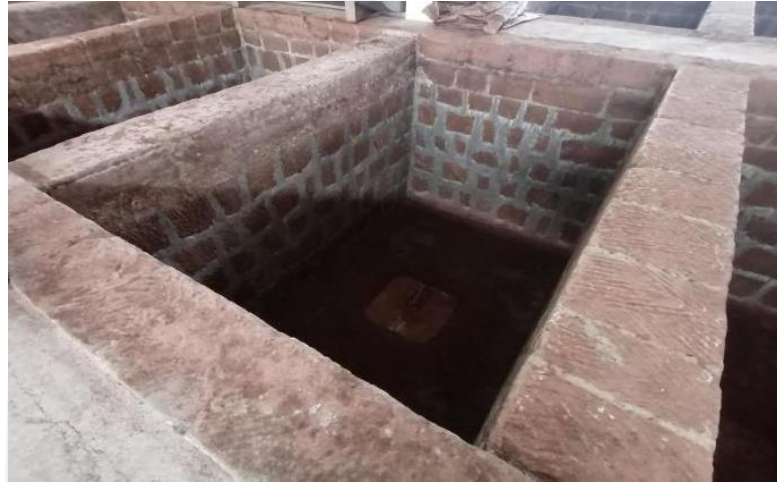
Figure 30 Moutai liquor cellar. The container of traditional Maotai-flavored wine is a stone cellar.
