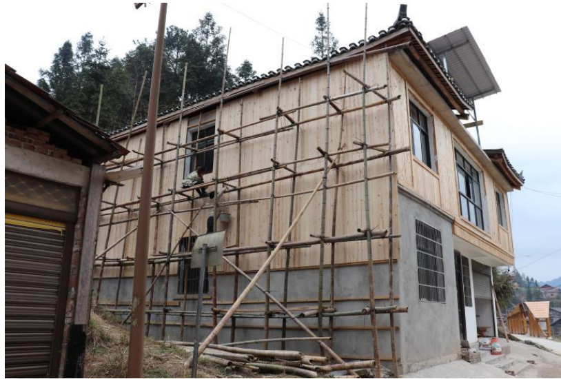
Figure 4. 19 Houses under repair in Zaidang Dong village
