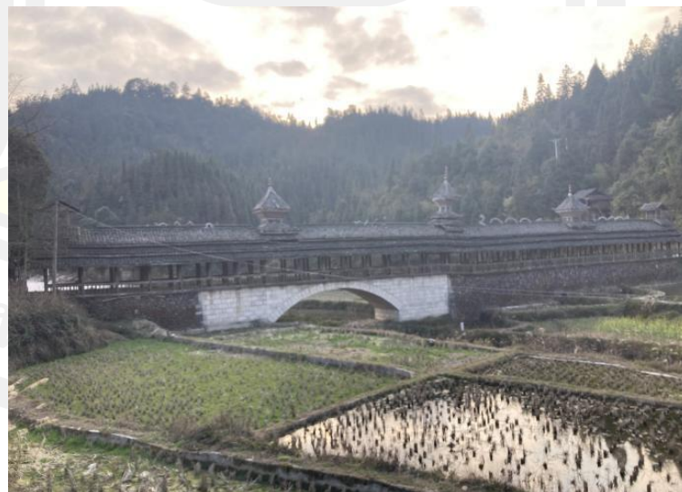
Figure 4. 3 The "Fengyu Bridge" across the mountains
