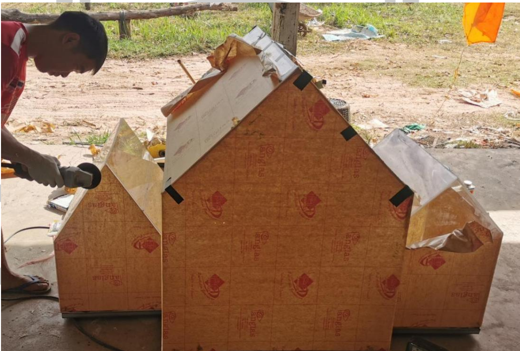
Figure 29 Work in step 4
