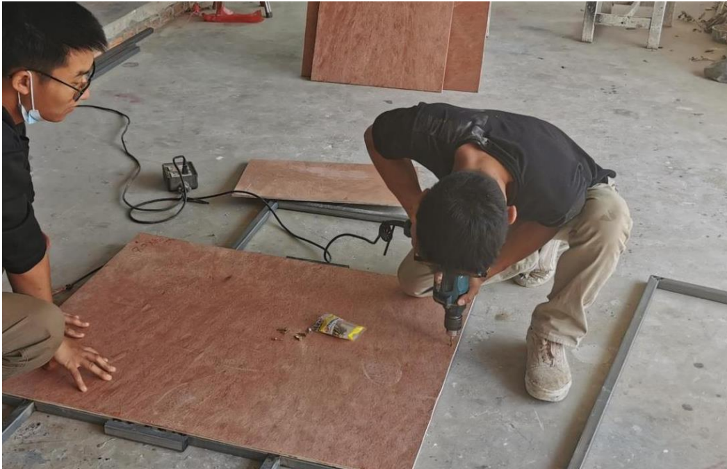
Figure 26 Work in step 1
