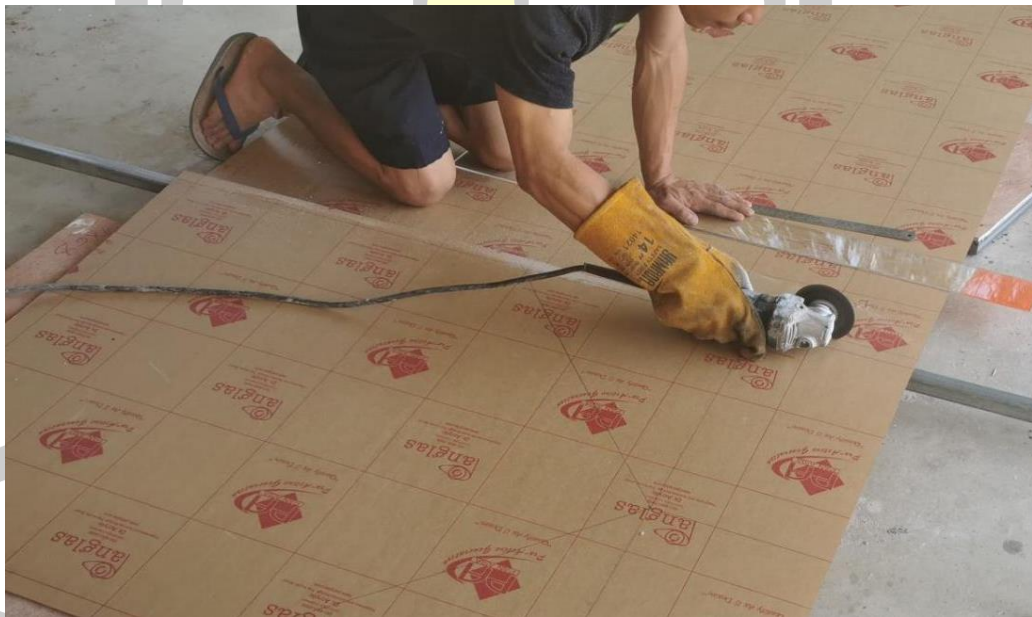
Figure 27 Work in step 2
