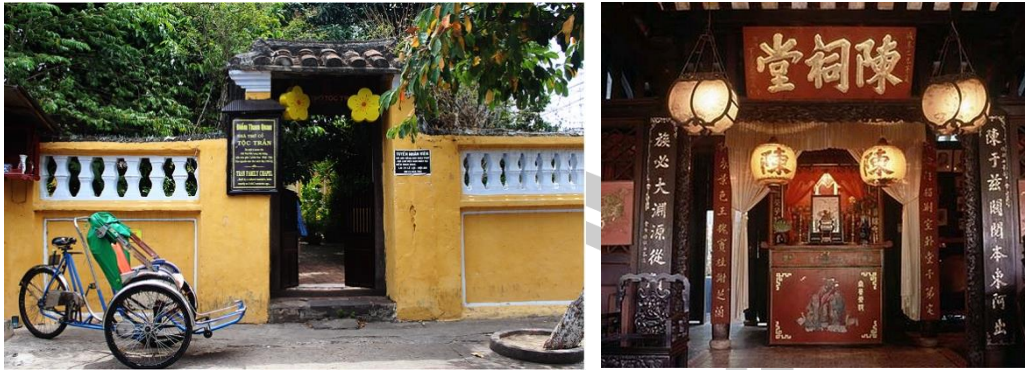
Figure 13 Church of the Tran family on Tran Phu - Hoi An street Source: Nguyen Thi Thanh Thao (May 22, 2022)
