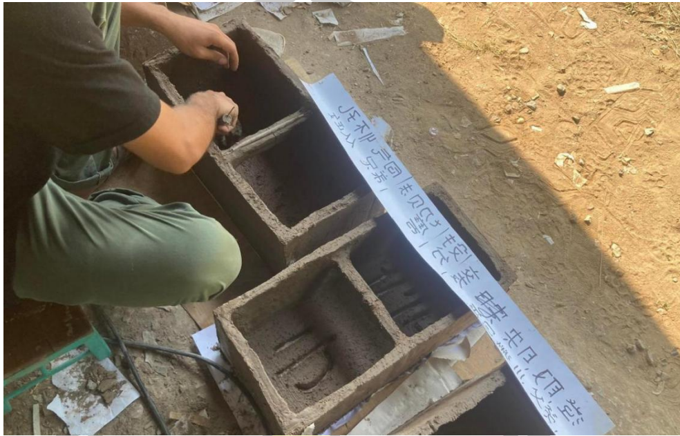
Figure 17 Work in step 3
