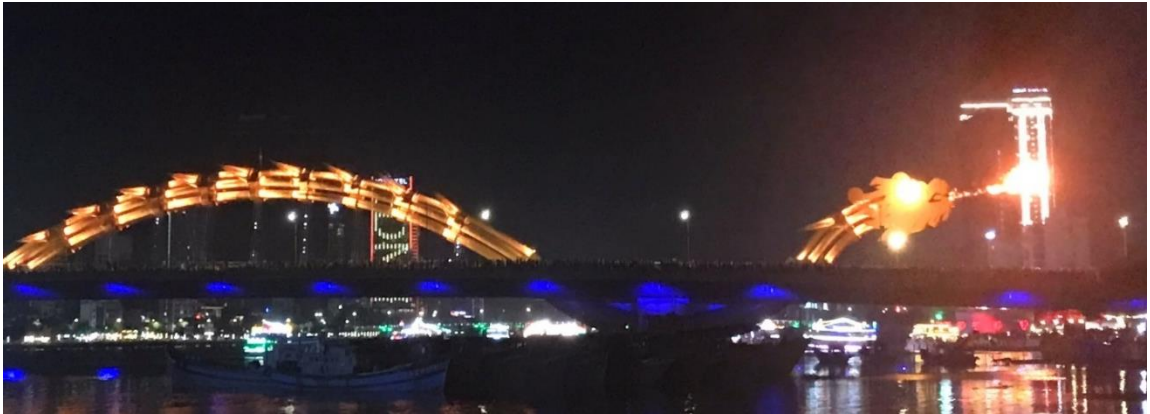
Figure 45 Dragon Bridge – Da Nang.
