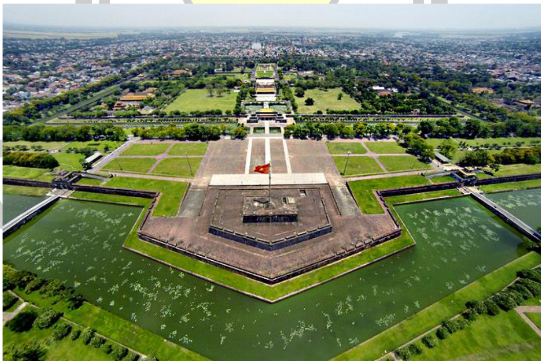
Figure 6 Panoramic view of Hue Citadel from above
