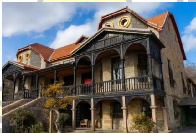
Figure 23 Siyan Building, Huancui District, Weihai City
