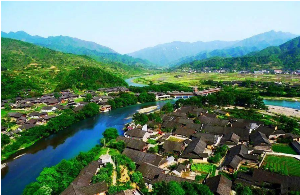
Figure 60 Jabala Ancient Walled City, which has become the largest Tujia group building in the country
