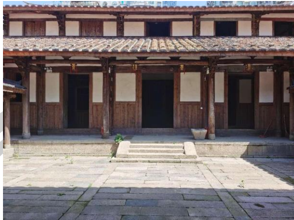
Figure 19 The hall of the grandparents is located in the middle of the third floor, which is the place to put the spirit seats of the ancestors. The two compartments on the east and west of the first floor are the rooms where the elders live, with the eldest elders residing in the east compartment and the youngest ones in the west compartment. Instead, the unmarried daughters had to go up through a narrow crawl to the second story in the attic.
