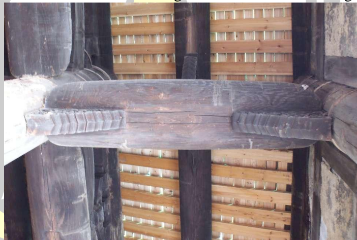
Figure 22: Cicada strand pattern on substitute wood
