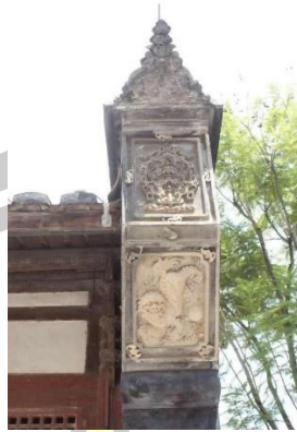
Figure 30 Plastered lion playing with a ball on the reading board of the gatehouse of the Chen Family Alcove.
