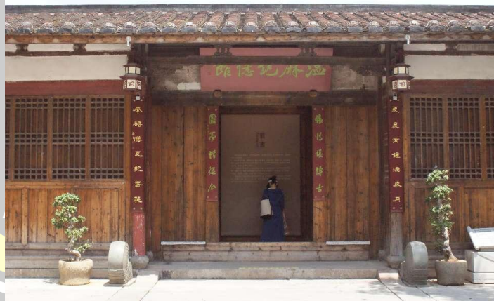
Figure 29 The gatehouse of the Chen Family Alcove reflects the characteristics of a merchant's building used for both commercial and residential purposes.
