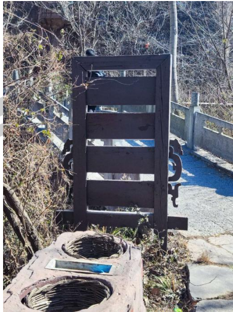
Figure 29 Status of some of the signage in the Longtan Grand Canyon scenic area in Luoyang
