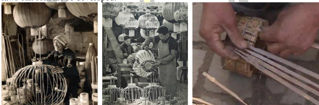
Figure 44 Red gauze lanterns before the reform and opening up, with a skeleton made of bamboo gimlets and wooden upper and lower seats
