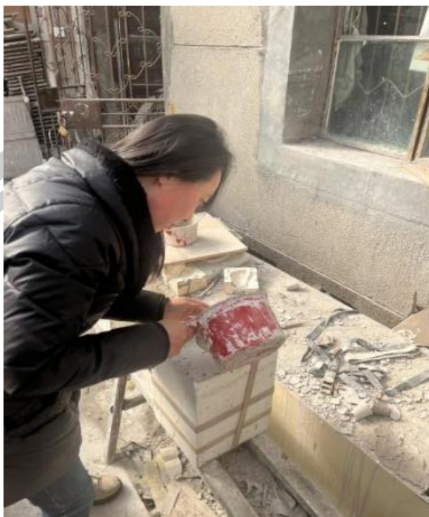
Figure 127. Use a plaster mold for grout Source: Photography by Zhang Lin, 2023
