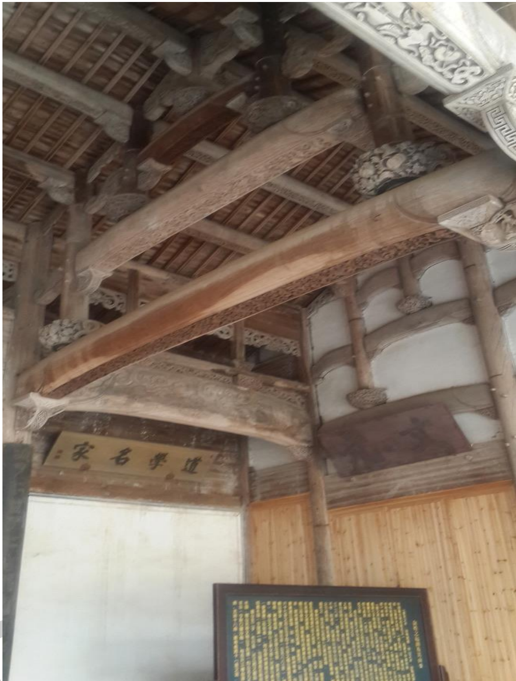
Figure 110 The beam frame of Yu's ancestral hall in Wangkou Village, Wuyuan County
