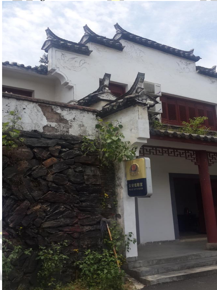
Figure 31 "Horse Head Wall", one of the important features of Wuyuan Huizhou architecture
