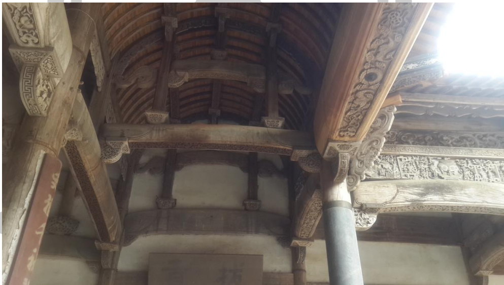
Figure 67 The brackets and carvings of the Yu Ancestral Hall in Wangkou Village, Wuyuan Image source: Hu Yu, taken on May 26, 2017, in Wuyuan County, Jiangxi Province.
