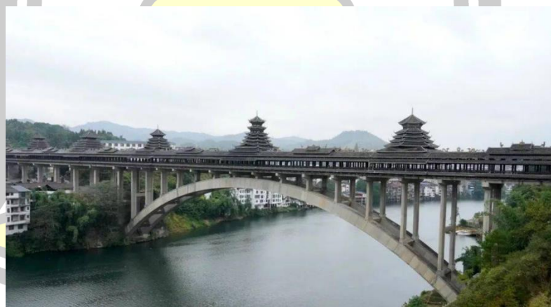
Figure 105 Longji Wind and Rain Bridge in Sanjiang County. It is the longest wind and rain bridge in the world in terms of length and scale. It can be used for traffic in the middle and pedestrians on both sides. It is a model of a modern wind and rain bridge. Source: https://travel.sohu.com/ (Accessed on March 26, 2024)
