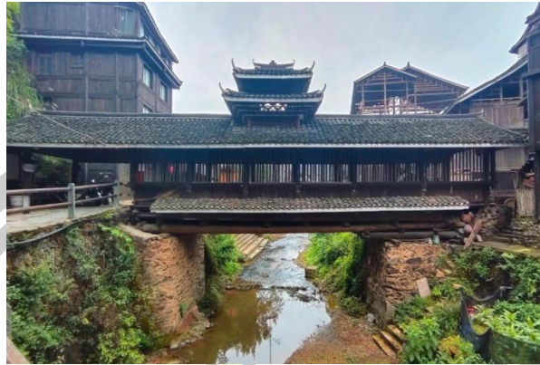
Figure 21 Pin'an Bridge without piers. The Pin'an Bridge is 23.5m long, has a small span, and has no piers. It uses wooden beams as the bridge span and is directly erected on the stone abutments on both sides. Source: Photographed by Chen Lu. May 2, 2023
