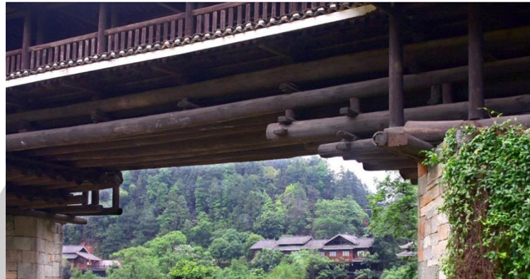
Figure 43 The span of the Yongji Bridge. It uses an outrigger beam structure, which increases the span of the bridge and evenly concentrates gravity on the piers and abutments, increasing the support area. This bridge support method is the local wisdom of the Dong people in building bridges. Source: Photographed by Chen Lu. May 1, 2023
