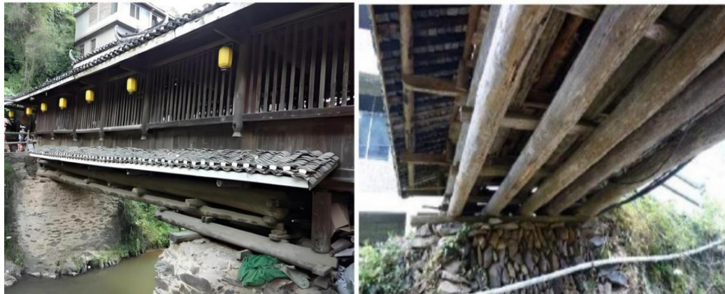
Figure 22 The span of the Pin'an Bridge. It adopts a simply supported beam structure. The simply supported wooden beam structure is common in small-scale wind and rain bridges. Source: http://image.baidu.com/ (Accessed on March 10, 2024)
