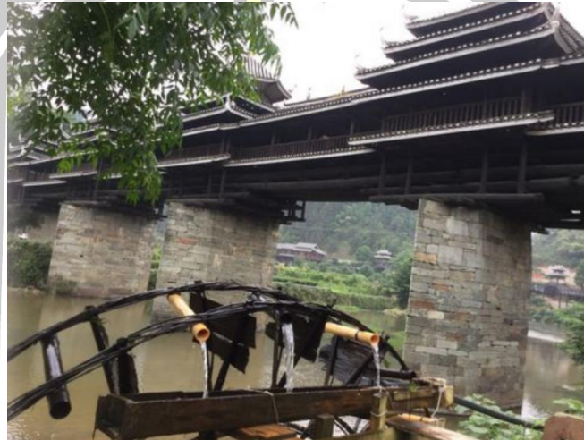
Figure 44 The pier of Yongji Bridge. It is a six-sided cylinder made of bluestone. This shape can reduce the impact of water flow and increase the support stability of the pier. Source: Photographed by Chen Lu. May 1, 2023
