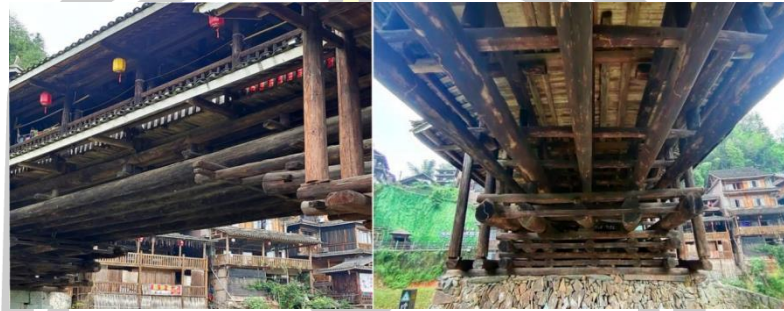
Figure 23 The span of the Helong Bridge. It adopts an extended-arm wooden beam structure. The extended-arm wooden beam structure can increase the support area and is often used in wind and rain bridges with larger spans. Source: http://image.baidu.com/ (Accessed on March 10, 2024)
