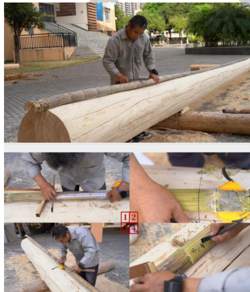
Figure 34 The process of making craft poles by Mr. Yang Yunqing, a Dong carpenter. He first scraped the bamboo skin and then used a ruler and pen to write the length and size of the building components on it with ink. When writing the names of various parts of the house, he used the unique "moshi" Character. Source: Photographed by Bian Jishen. December 26, 2022
