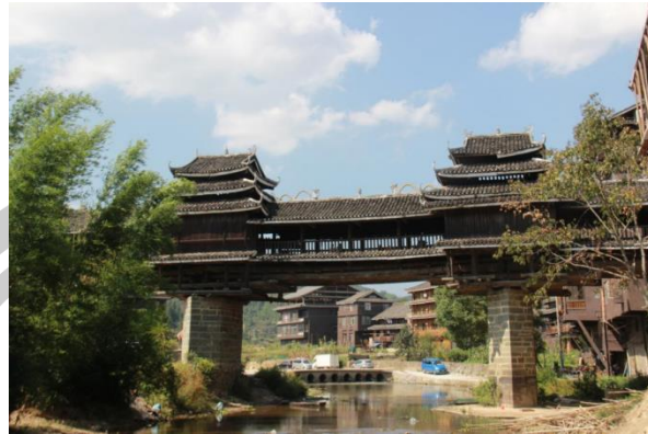
Figure 20 Piers of Puji Bridge. Puji Bridge is located on the Linxi River. The bridge is 51.4 meters long and has a large span. Bluestone piers are built in the water to support the bridge. The bridge piers are hexagonal, which can effectively resist water flow. Source: Photographed by Chen Lu. May 2, 2023
