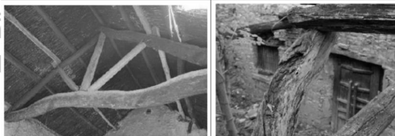
Figure 86 Timber damage types Source: Photographed by author, May 25, 2020
