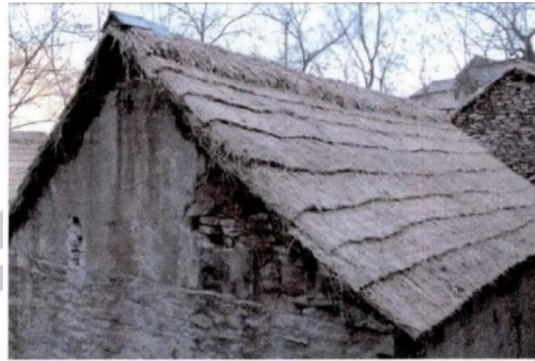
Figure 46 Thatched roof house. The roof covering material is made from yellow grass that is commonly found in the area. Source: Zhang Xiaonan "Research on the Regional Characteristics and Construction Techniques of Traditional Stone Residences in the Mountainous Areas of Central Shandong" (Accessed on February 29, 2023)
