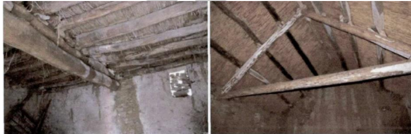
Figure 41 Roof truss structure Make full use of natural resources in the mountains to build. Source: Zhang Xiaonan "Research on the Regional Characteristics and Construction Techniques of Traditional Stone Residences in the Mountainous Areas of Central Shandong" (Accessed on February 29, 2023)
