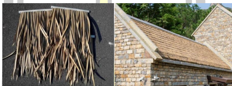
Figure 89 Simulated thatched roof. The roof effect has been restored to its traditional appearance through modern materials and technology. Source: Photographed by author on June 7, 2023
