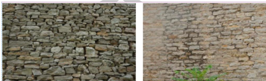
Figure 43 Types of stone wall masonry construction methods for stone houses. The stones built by wealthy families are large and regular in size. They rely on the friction between the stones to dry-lay and are used to add facades to the front facade of the house. However, the masonry stones of homes with average economic conditions are relatively messy, and small stones or slurry are usually used to fill the gaps after masonry. Source: Song Wenpeng "Research on Spatial Form of Traditional Villages in Shandong" (Accessed on July 18, 2023)
