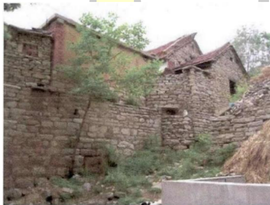
Figure 40 Building platform. The platform base and the courtyard wall are integrated, and the man-made buildings and the natural environment coexist harmoniously, which is a reflection of local wisdom. Source: Zhang Xiaonan "Research on the Regional Characteristics and Construction Techniques of Traditional Stone Residences in the Mountainous Areas of Central Shandong" (Accessed on February 29, 2023)
