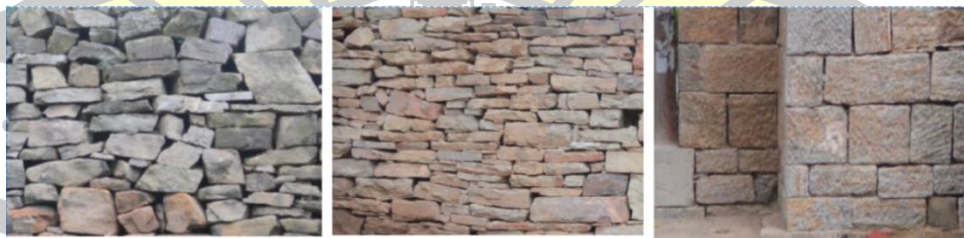
Figure 42 Stone types. The random rough stones are of different sizes, laid freely horizontally and vertically, with gravel caulking and dry-laying; the flat rough stones are of equal size, laid horizontally and bonded with clay; the striped stones are large and regular, with staggered seams and overlapping joints, and are arranged in an orderly manner. Dry build. Source: Zhang Xiaonan "
