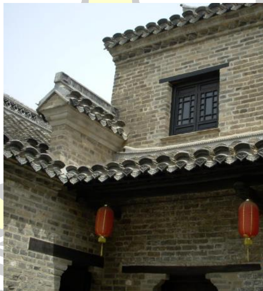
Figure 76 The dripping shape of tiles in ancient houses in Yaowan Ancient Town Source: Photographed by Peng Bao, 2021
