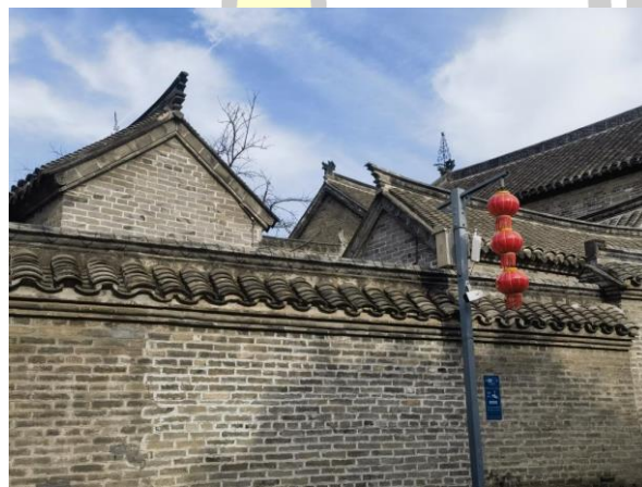
Figure 71 Xuzhou's ancient houses basically use hard gables Source: Photographed by Peng Bao, 2023
