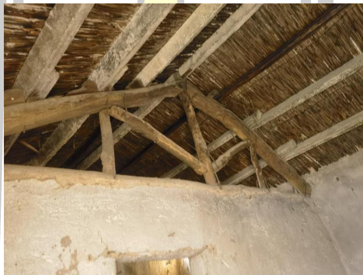
Figure 53 Fence material rooftops of ancient houses in Zhakou Village
