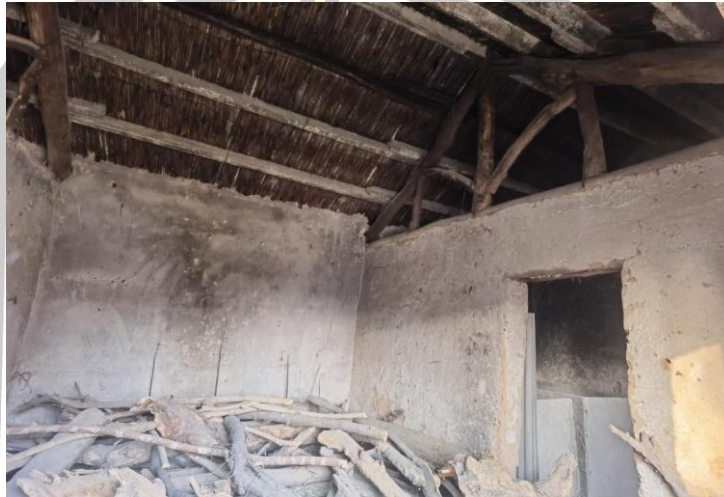
Figure 73 The wooden beam structure in ancient Xuzhou only used a quarter of the wood from other regions.
