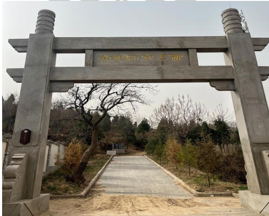
Figure 18. Entrance to the site of the Xihan Imperial Granary
