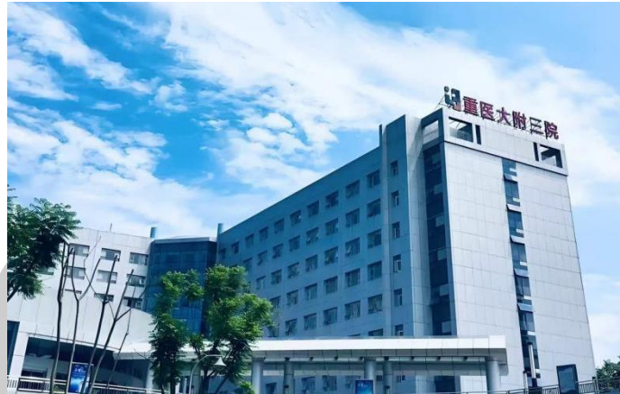
Figure 17. A City Hospital in Chongqing
