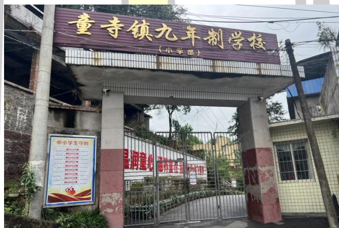
Figure 119. Fushun County Tongsi Town Nine-Year School (Tongsi Primary School)
