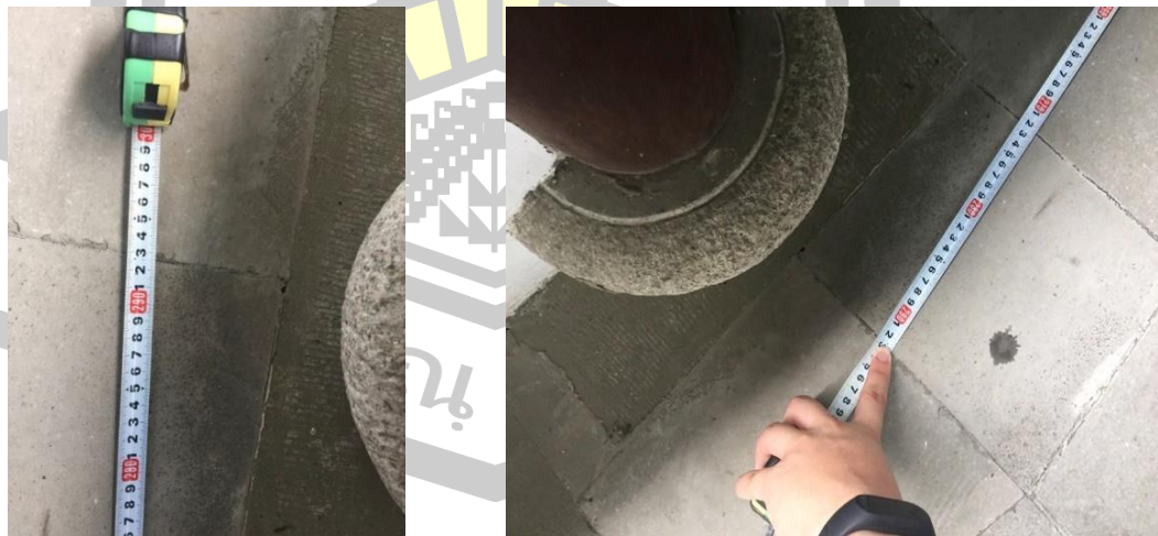
Figure 103 The bottom of the gallery is measured
