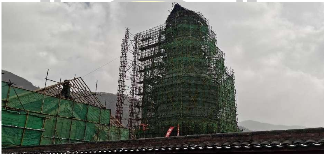
Figure 35 Ancient buildings under repair
