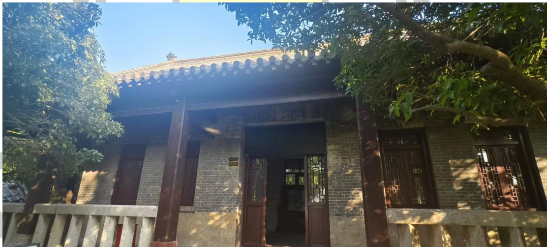
Figure 15 The Fanghe Pavilion Photos Source: Photographed by the author (2024)
