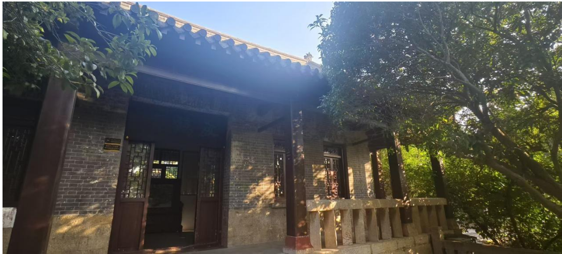
Figure 16 The Fanghe Pavilion Photos Source: Photographed by the author (2024)
