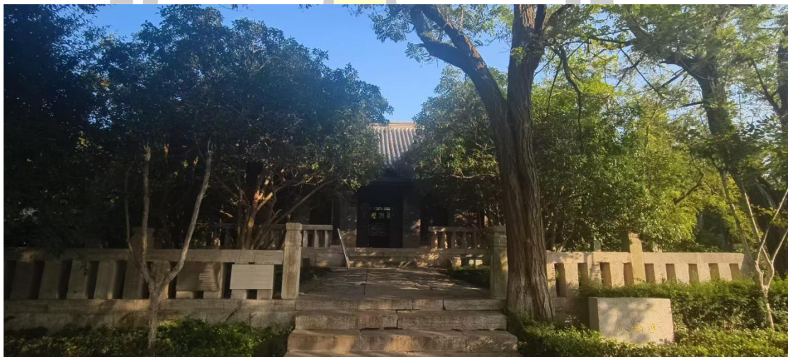
Figure 17 The Fanghe Pavilion Photos Source: Photographed by the author (2024)
