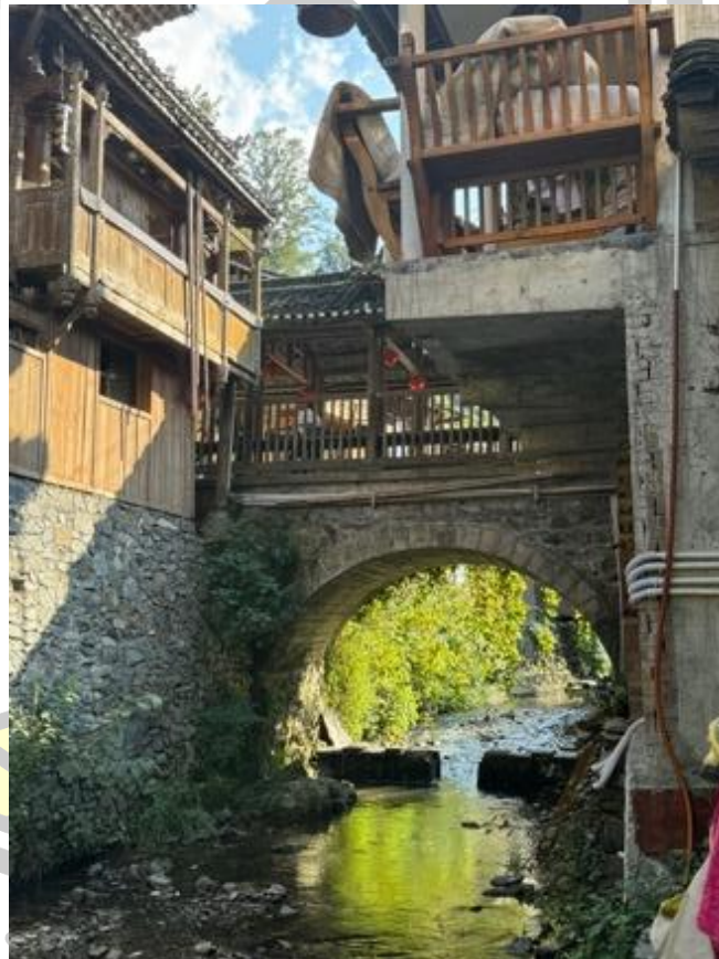
Figure 15 The first wind-and-rain bridge in Dali Village, which is close to the highway entrance
