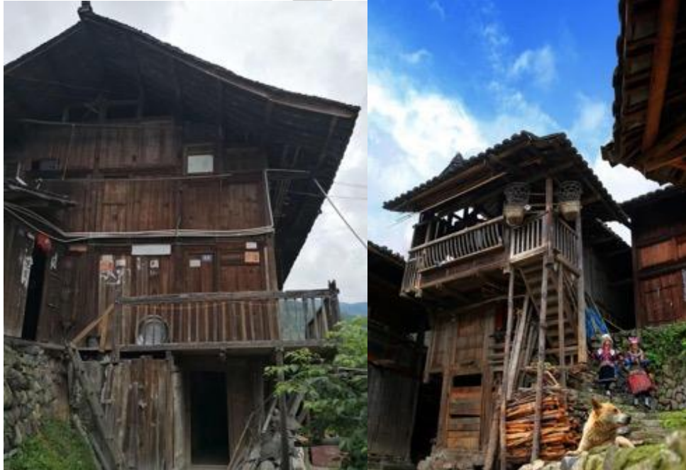
Figure 6 Stilted wooden house (diaojiaolou) in Miao Village Source: Ziyi Ye (2022)
