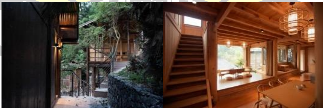
Figure 60 The renovated homestay provides a more modern interior space for foreign tourists. Exterior space (left), interior space (right) Source: Wuming Architecture Studio (2023)
