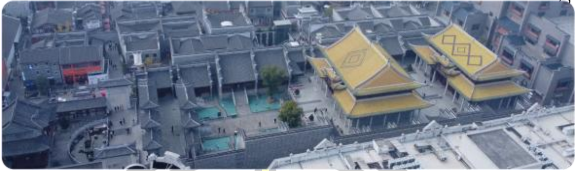
Figure 19 Aerial view of Wanshou Palace Historical and cultural Block
