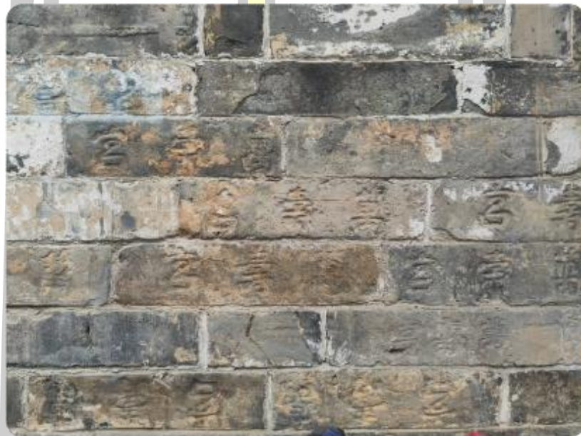
Figure 73 A display of building bricks engraved with the word "Wanshou Palace"
