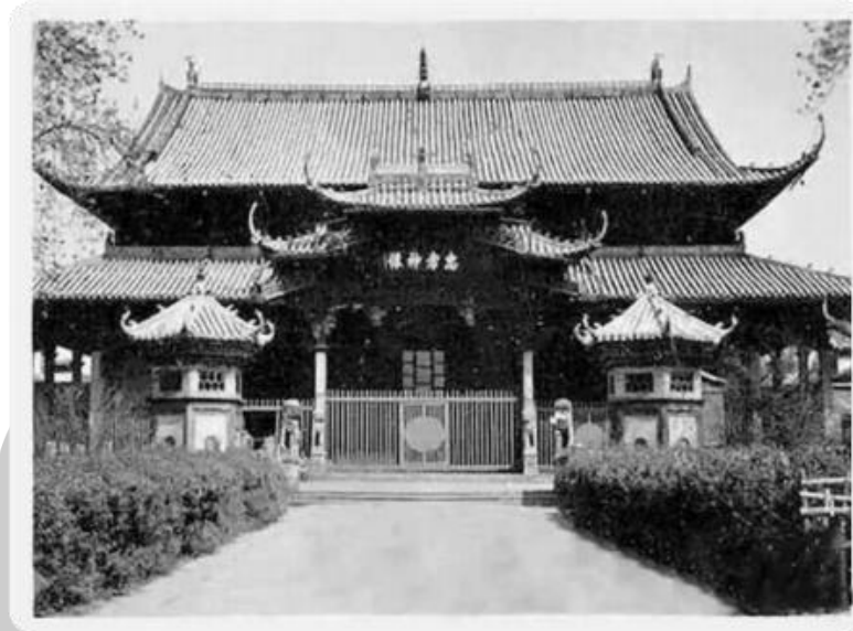
Figure 32 Photographs of the reconstruction of Wanshou Palace in Nanchang during the Republican period in 1915
