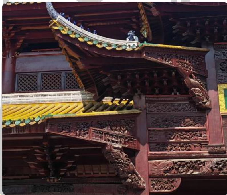
Figure 37 Wood carved dragon ornament at the eaves corner of the Zhenjun Palace
