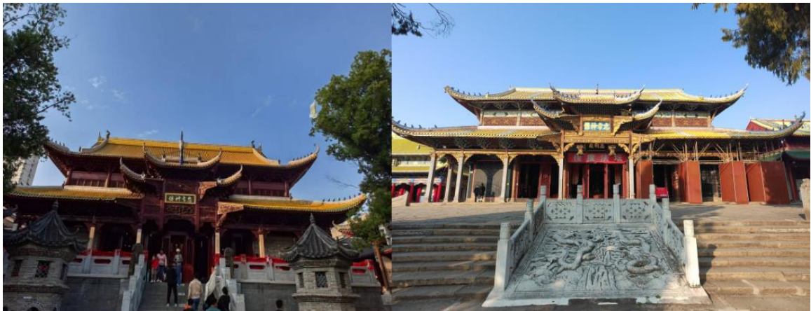
Figure 71 Tiezhu Wanshou Palace Zhenjun Palace Reenactment of the Xieshan Mountain Summit Architectural Style(left) Xishan Wanshou Palace Gaoming Palace Reenactment of the Xieshan Mountain Summit Architectural Style (right)
