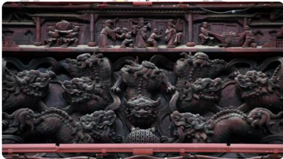
Figure 62 The architectural carving of the Tiezhu Wanshou Palace, which shows the exquisite carving technique using the traditional Chinese motif dragon, and the traditional Chinese story is carved above the dragon
