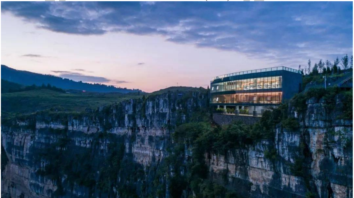
Figure 50 Karst Art Museum (located on a huge rock wall built on the north side of Haiwei Valley in Anlong, Guizhou, offering a panoramic view of the entire valley, including peculiar peaks, strange rocks, rivers, and Tiankengs)
