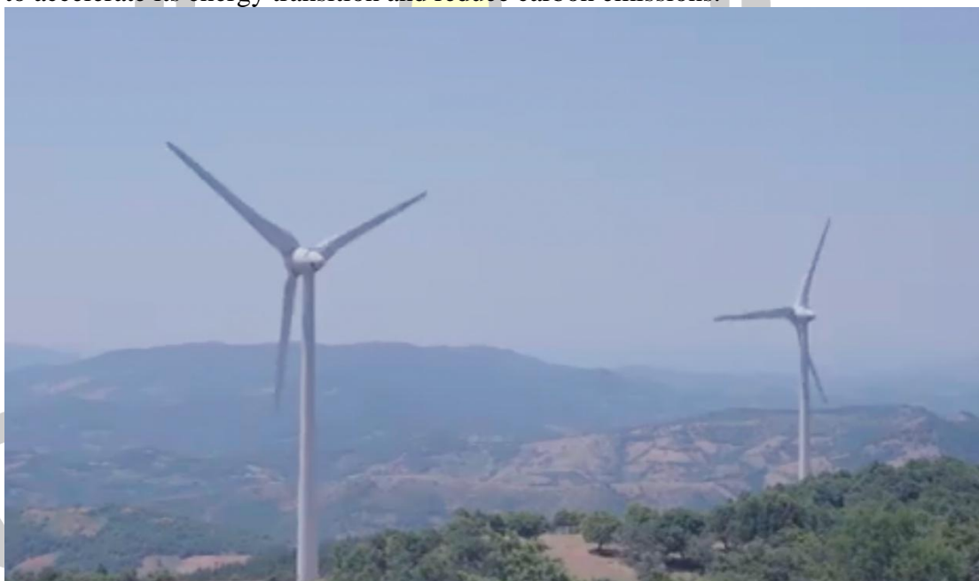
Figure 44 The Thrace Wind Power Project in the Belt and Road Process.
